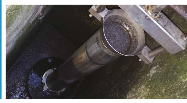
A hydrostatic telescopic bellmouth would usually be fixed directly to desludging pipework via a flanged connection, however, on this occasion, no such flanged connection was available as the existing bellmouth was cast into the chamber floor in this part of the sewage works.
