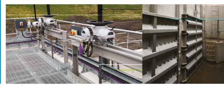
IBS' RPS range of penstocks was chosen, as this design offers excellent performance and durability, with added features such as a unique door stiffener design, which alleviates the risk of crevice corrosion due to the trapezoidal shape and drainage slots.
